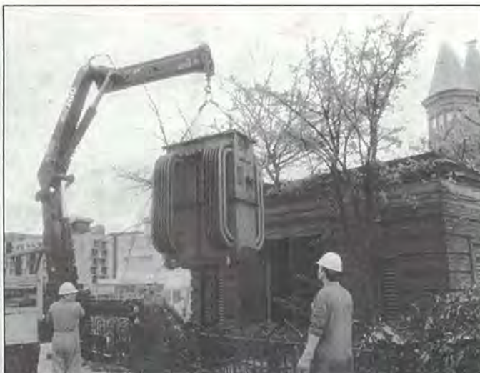
Members of Liverpool District's fitting team remove the transformer from the London Road substation. At the Hiab controls is driver Bill Harrison with Mike Byrne (centre) and Les Dolan.
