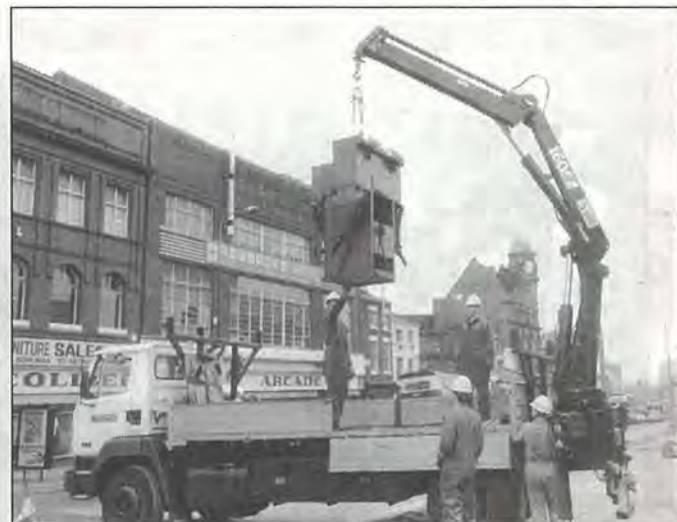
Up, up and away. The redundant switchgear is loaded onto a Manweb truck.
